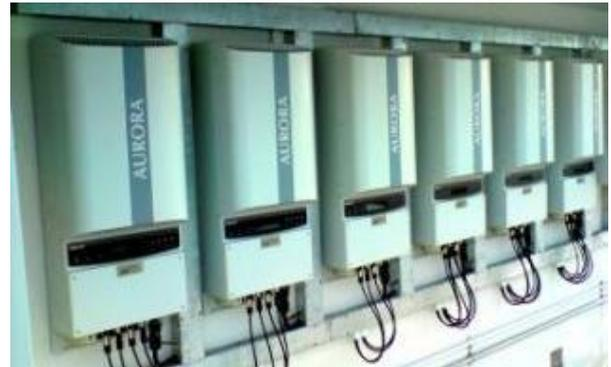
Figure 4. Inverters used in the PV system
