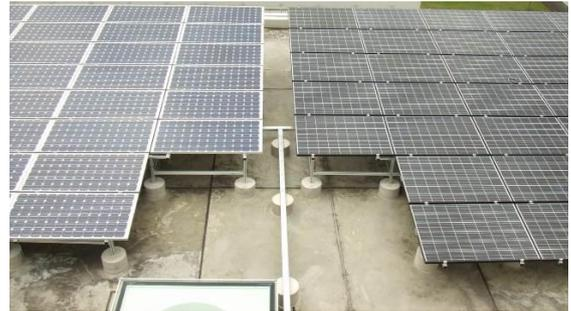
Figure 3. Picture of the 30.05kWp PV system installed on the rooftop of a 7 storey building
