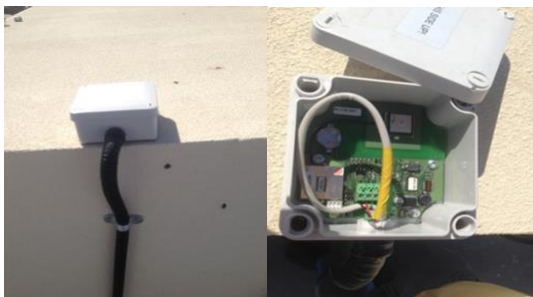
Figure 4:GPS installation at the roof
