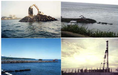
Figure 6: The beginning of land reclamation within Manado Bay in 1991 (Photos taken by Anton, 1992)
